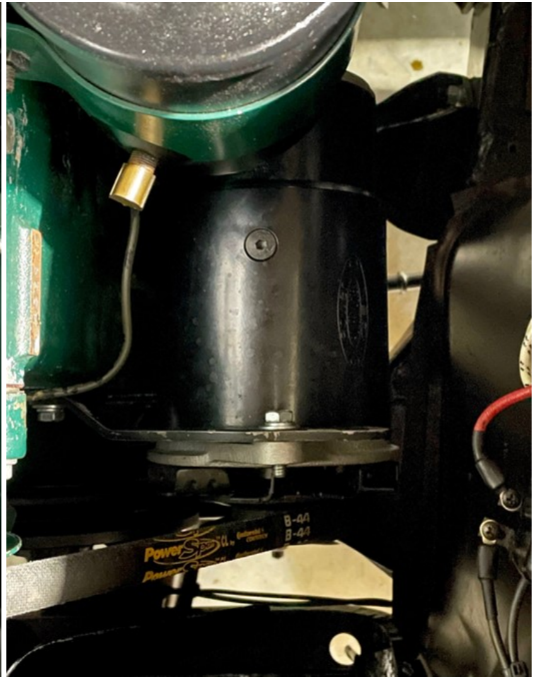
It was very tight fitting the new 12 volt Alternator in the housing of the generator, which was made in USA.
